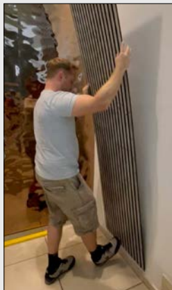
Mount the panels on the wall and adjust them.
