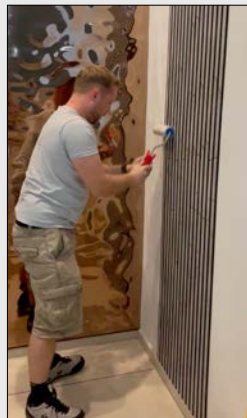
Press or roll the panel firmly into place. Tip: For secure fixing, use 2 to 4 screws.
