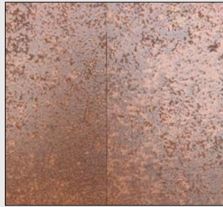
Processing without expansion joints
